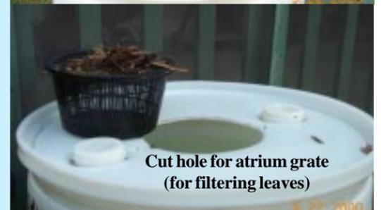
Cut hole for atrium grate (for filtering leaves)
