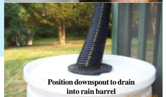
Position downspout to drain into rain barrel
