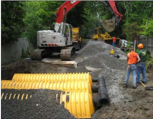
***Installing stormwater infiltration Chambers under the beach***
