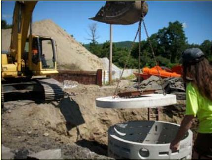
In the summer of 2010, the Warren County SWCD and Town of Lake George Highway Department completed a significant stormwater infiltration project at the town's highway facility. This system was designed by the District and treats all stormwater runoff from the totally impervious 2+ acre town highway property, eliminating a huge source of sediment and pollutants flowing into the adjacent waterbody, West Brook.
