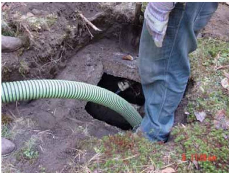
*Photo 9: Septic system pumpout and inspection*
